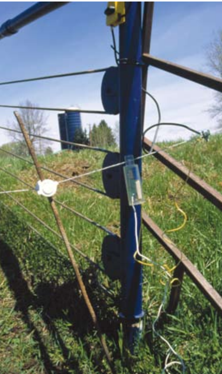
An example of smooth wire electric fencing.
