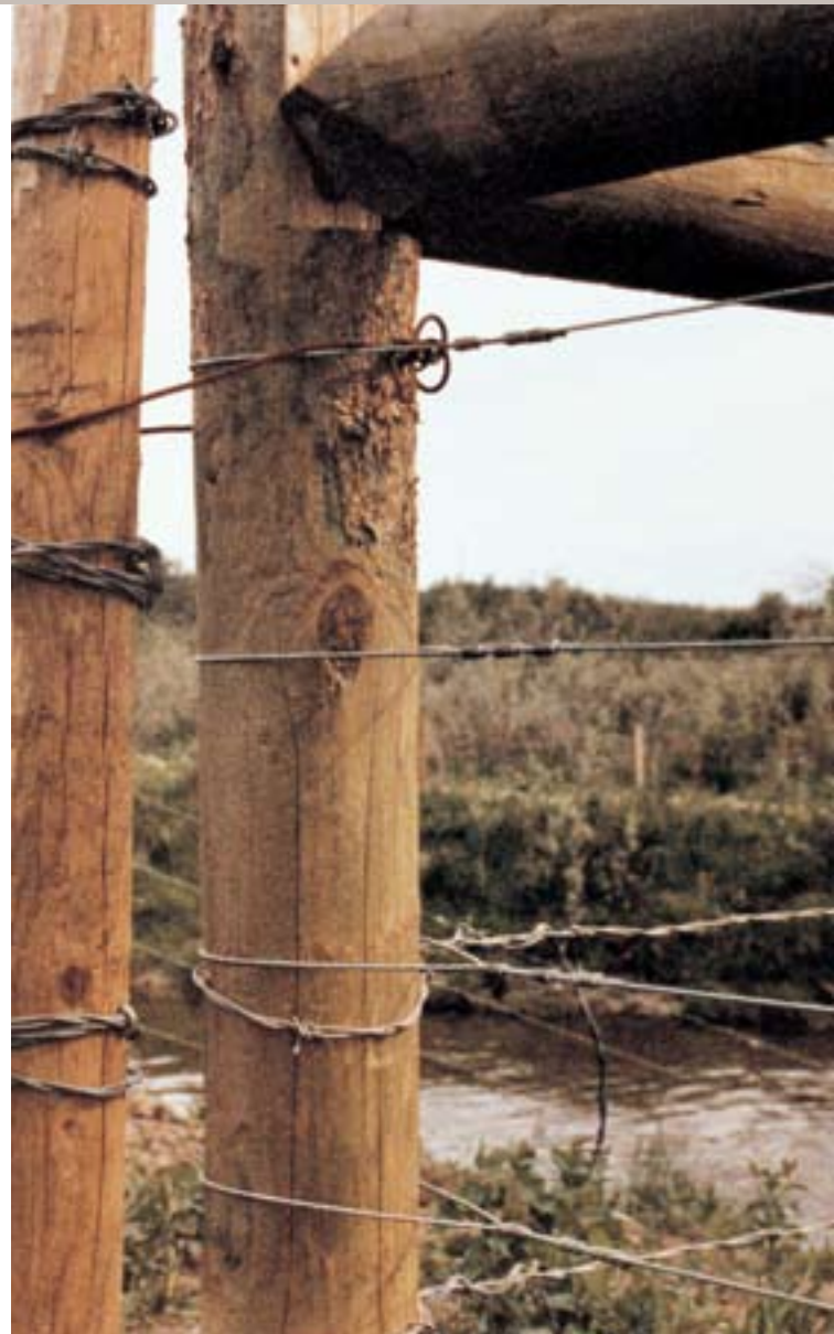
Corner post with high-tensile smooth wire and crimping sleeves.
